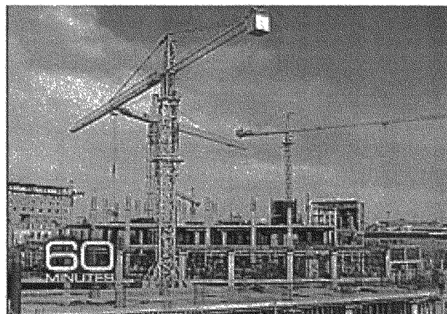
Construction in the Kurdish Iraqi city of Erbil (CBS)
