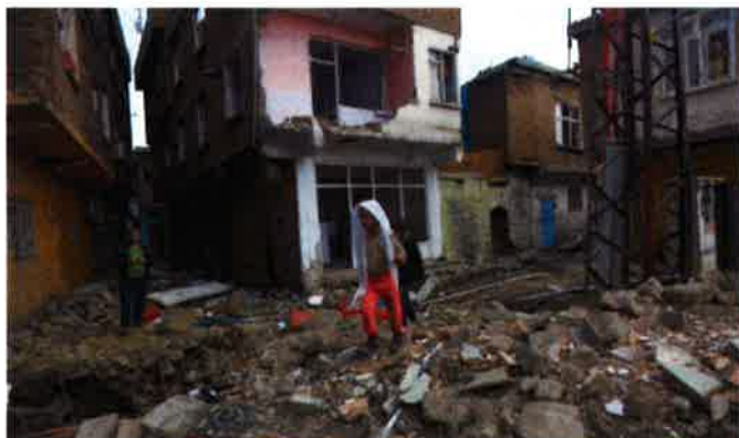
Children walk past by damaged buildings in Sur district, which is partially under curfew, in the Kurdish-dominated southeastern city of Diyarbakir, Turkey on February 19, 2016.
